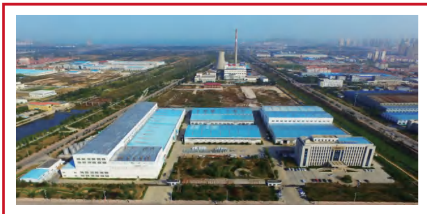
● Yantai Dongyuan Transformers Floor space: 150,000m 2
