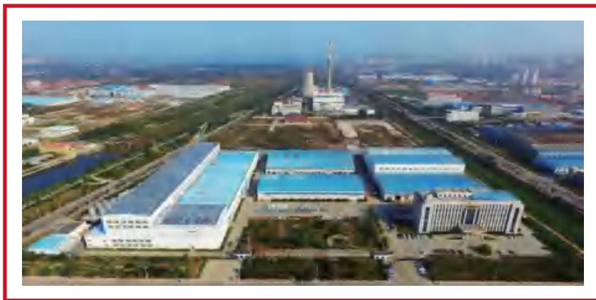
● Yantai Dongyuan Transformers Floor space: 150,000m 2
